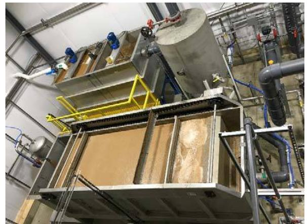
An automatic sludge transfer system with a level control device pumps the sludge from the sludge section into sludge holding tanks.
